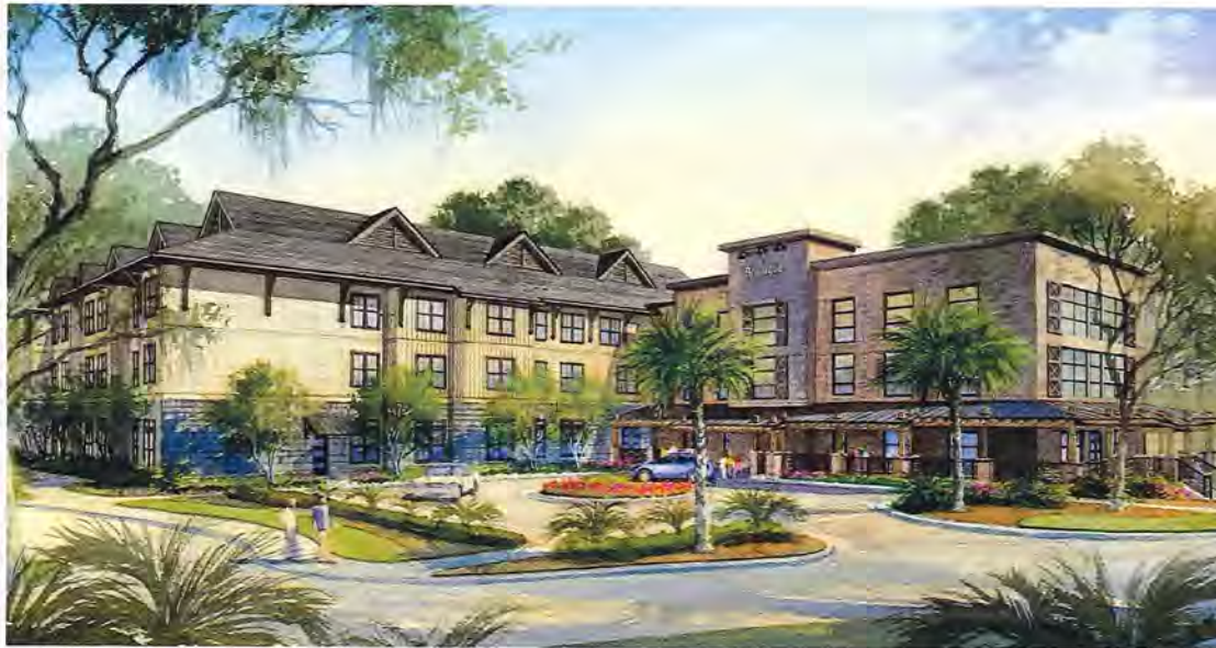
A rendering shows the three-story, 100-room Andell Inn that is currently under construction in South Carolina.
